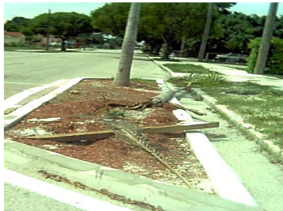
Vehicle-Caused Damage on Greenwood
