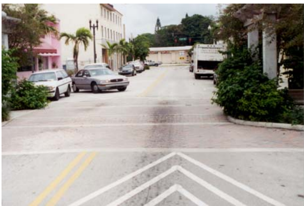
Nonstandard Chevron-Style Advance Speed Hump Markings on Northwood Road (Chevrons are normally placed directly
