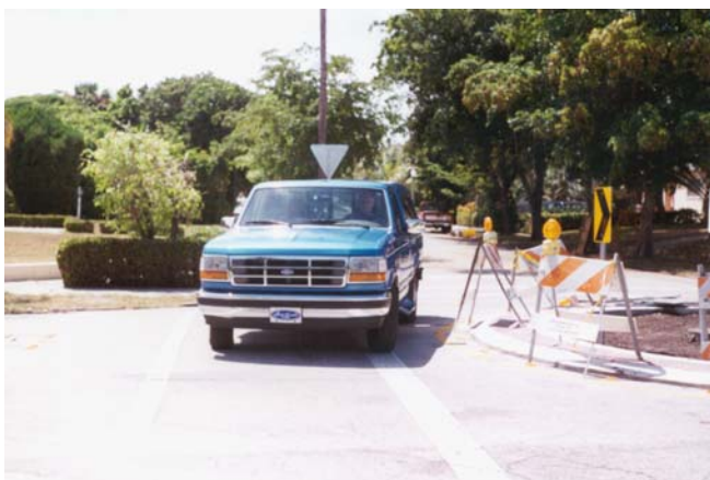
Vehicle is Forced to Drive in Crosswalk due to Roundabout
