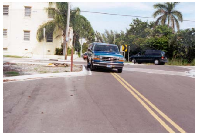
Vehicle is Forced to Drive into Opposite Lane by Neckdown
