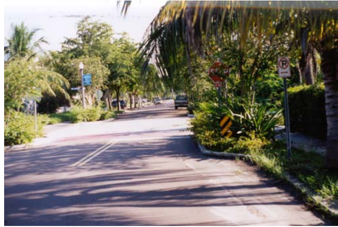
Stop Sign Obscured on Spruce Avenue Approaching 36 th Street
