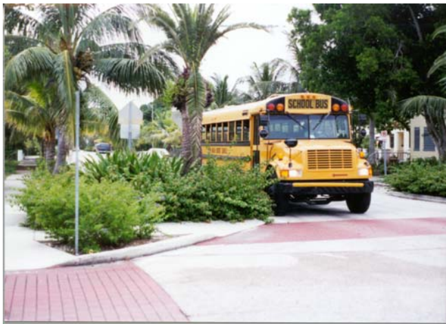
Overgrowth at 36 th Street and Spruce Avenue
