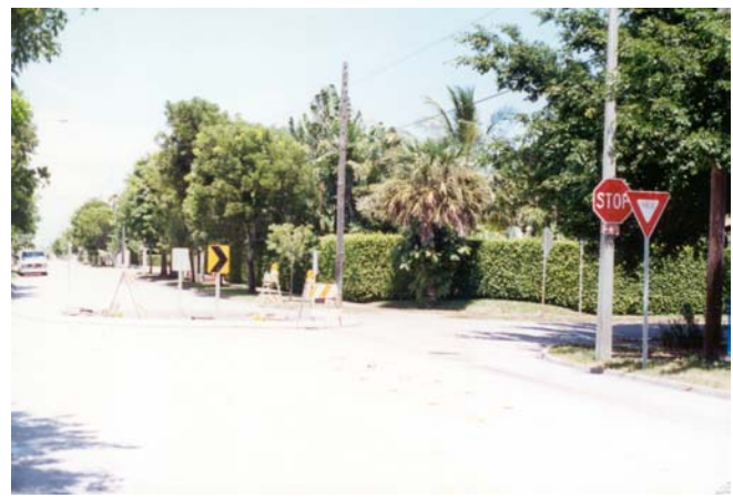
Conflicting Regulatory Signs on the Same Side of the Street
