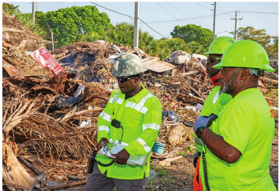
Assessing the debris field before work begins.
