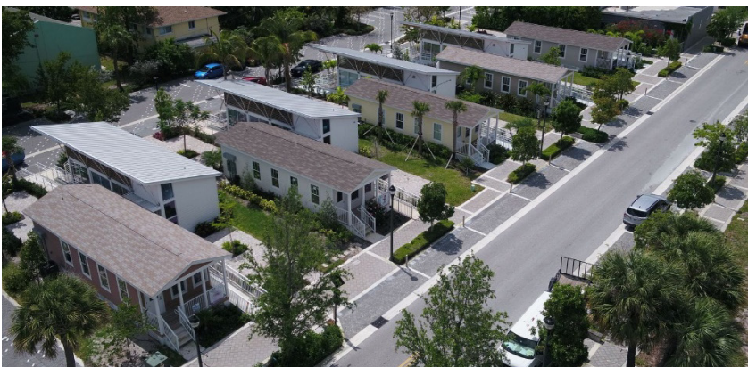
The Styx Historic Northwest
