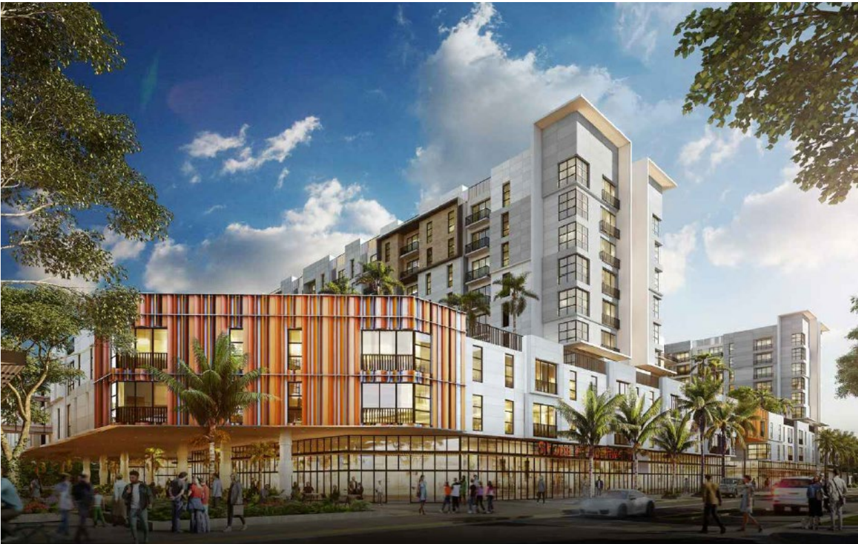
The District at Northwood (view from Broadway)
